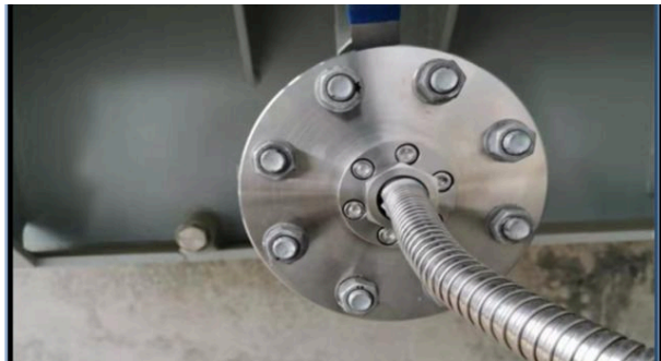
Field installation diagram of transformer oil valve type UHF sensor Field installation diagram of transformer external UHF sensor
