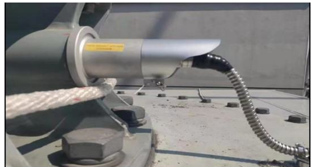
On-site installation diagram of transformer end-screen sensor
