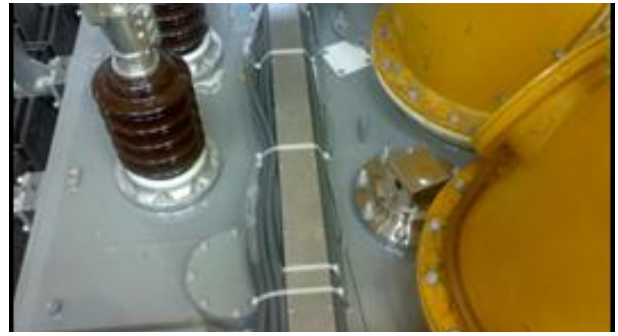
Installation diagram of the built-in UHF partial amp sensor on the transformer housing
