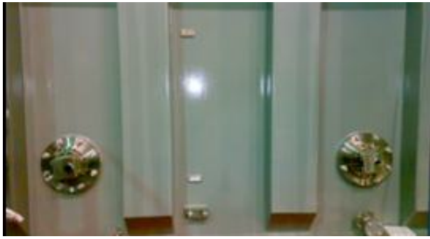
Installation diagram of the built-in UHF partial amp sensor on the transformer housing
