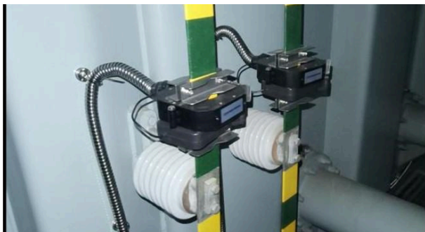
Field installation drawing of transformer core/clamp grounding current sensor Transformer RF sensor on-site installation drawing
