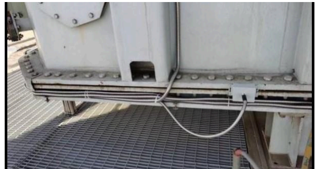
Field installation diagram of transformer oil valve type UHF sensor Field installation diagram of transformer external UHF sensor
